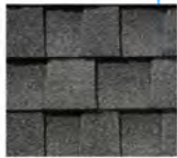
Architectural Asphalt Shingle Roof
