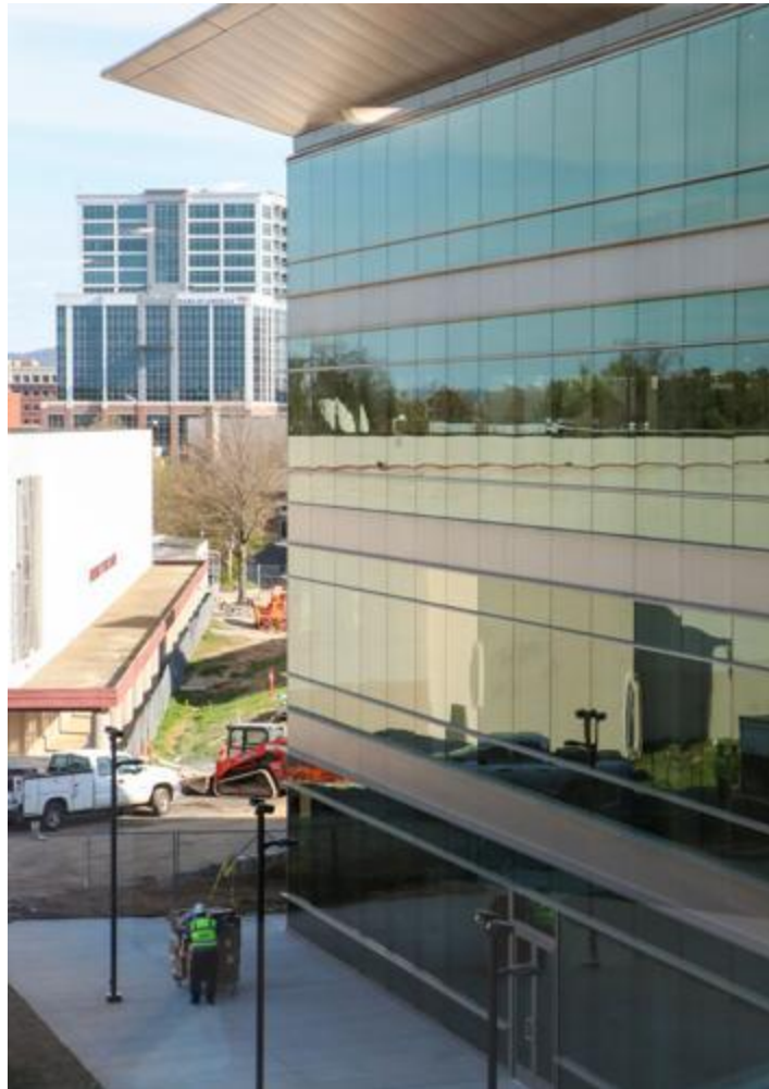
The new Greenville County Administrative Building. March 9, 2023.
