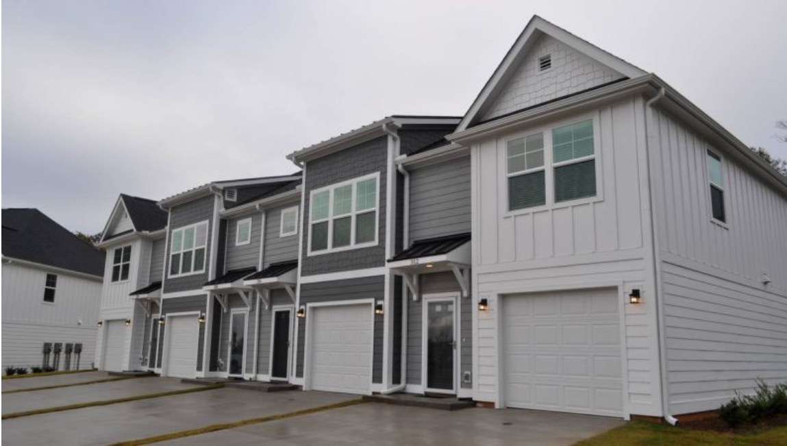
Fairview Townhomes on East Fairview Avenue in Greer consists of three buildings with 14 units. Photo by Megan Fitzgerald
