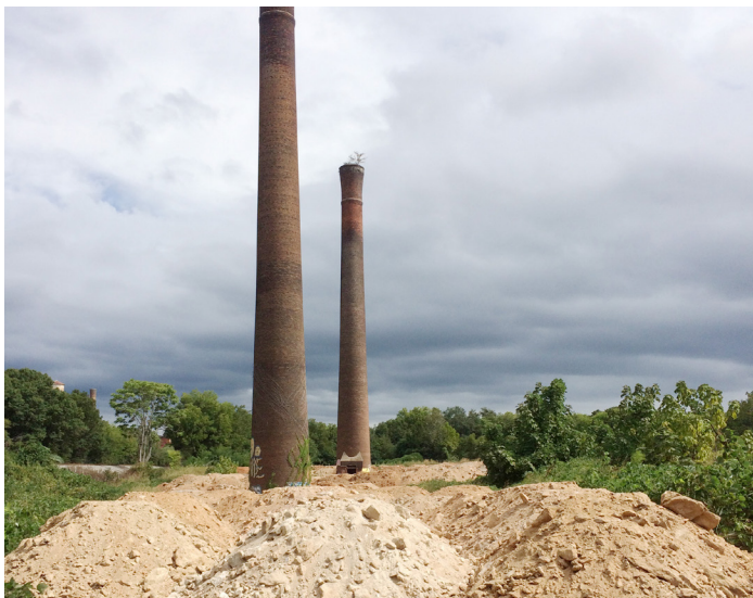
Former Poe Mill, Greenville
